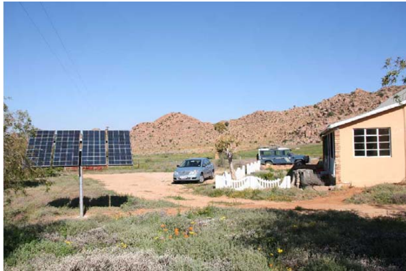
Large solar panels provide the research station with power.
