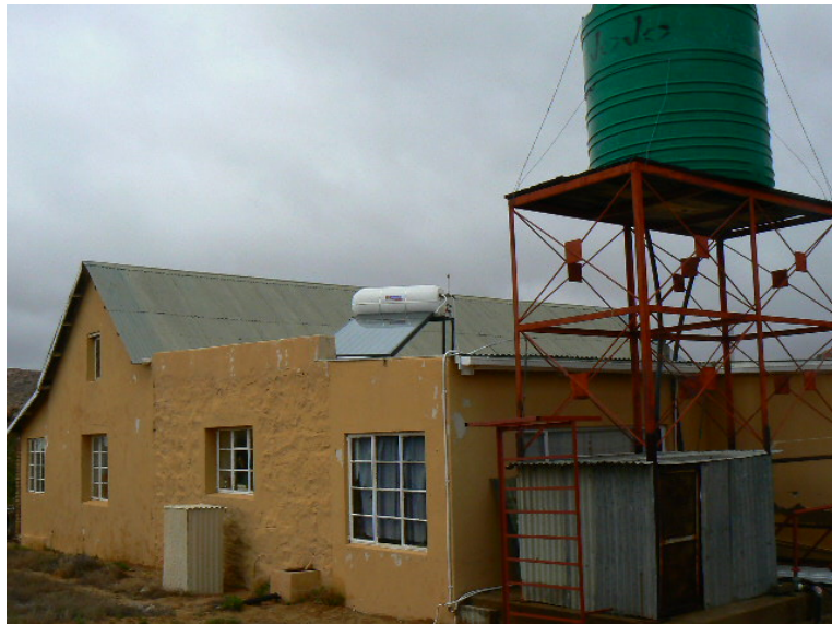
The solar geyser is placed on the roof of the research station.
