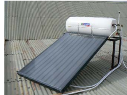
The new solar geyser can heat up 150 liters of water.
